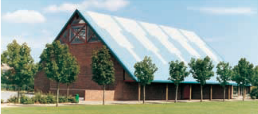
Exterior seen from the north west end (Photographer R.A. Brooks).
