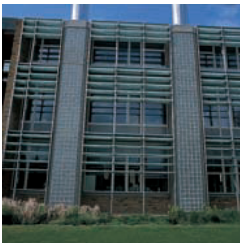
(c) Exterior of the south elevation showing the louvres (Photographer David Loe).
