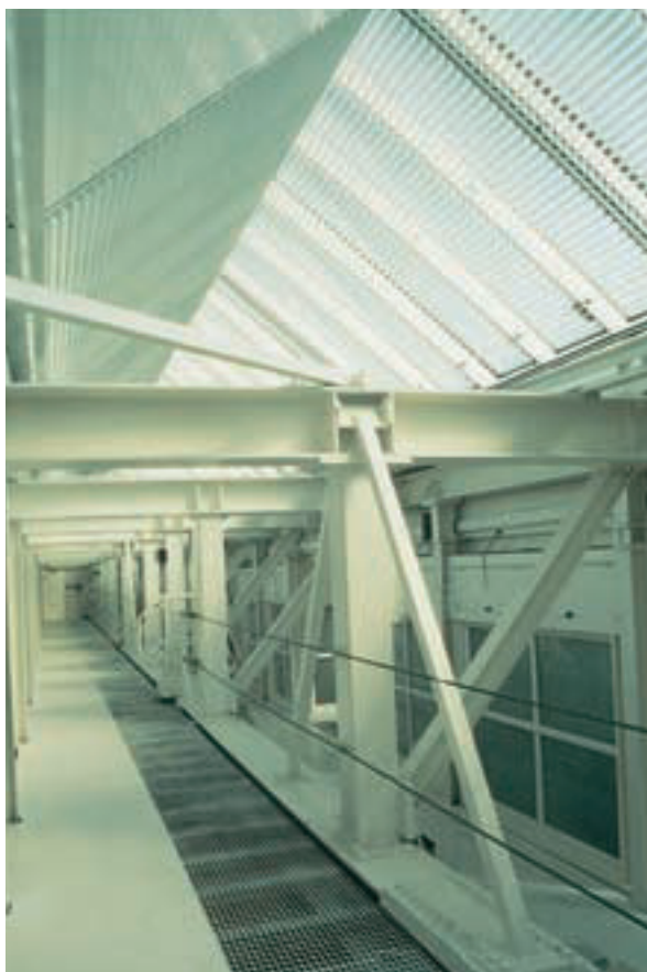
View at roof level showing daylight detail, with access to catwalks (Photographer David Loe).
