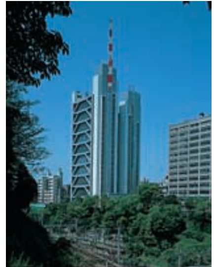
Exterior of the tower, day and night (Photographer Ian Lambot).
