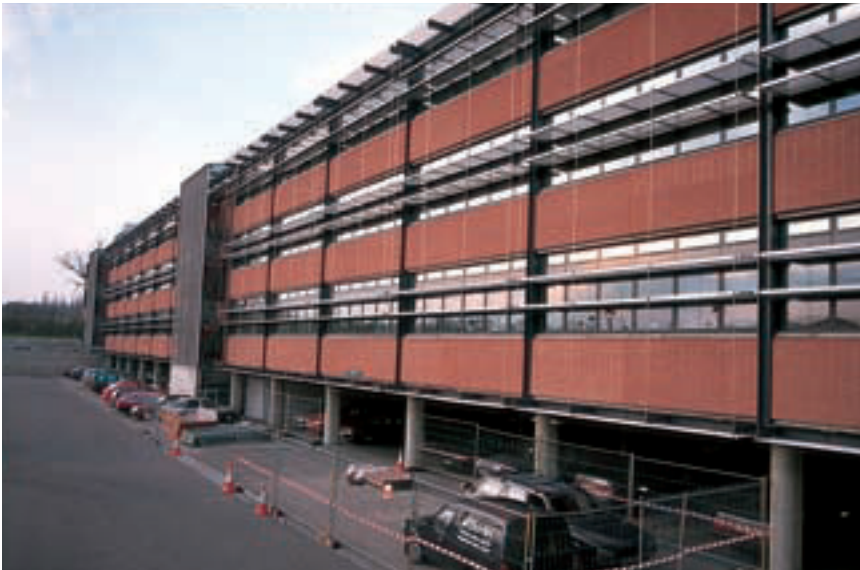
Exterior view of south elevation (Photographer Derek Phillips).
