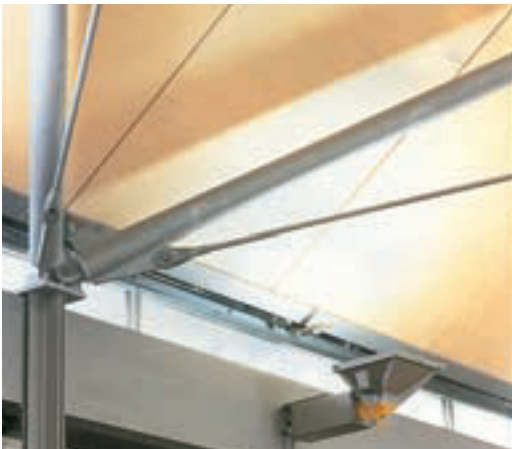
Detail of clerestory windows' structure and uplighter (Photographer Anthony Oliver).
