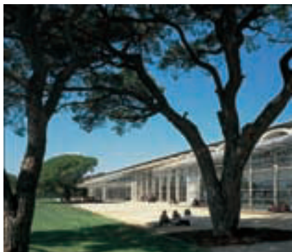
Exterior, north side (Photographer Dennis Gilbert).
