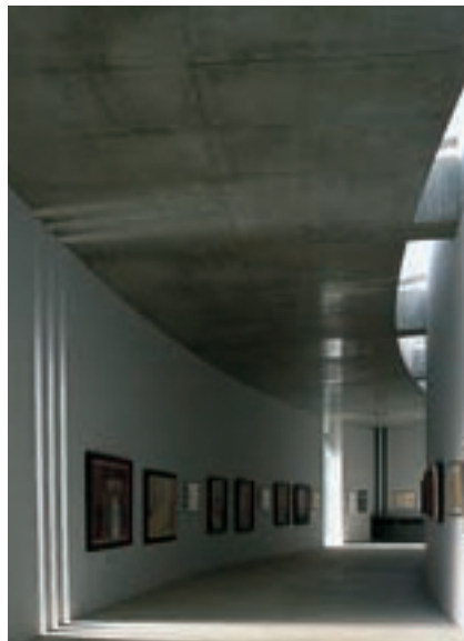
Interior of gallery showing the daylight slot (Photographer, Kaori Ichikawa, Tadao Ando).
