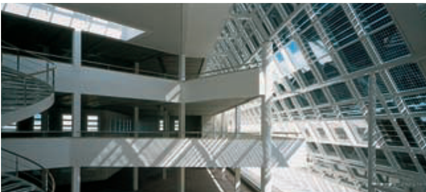
Interior looking towards the PV wall, showing the daylight effect (photography Studio E).
