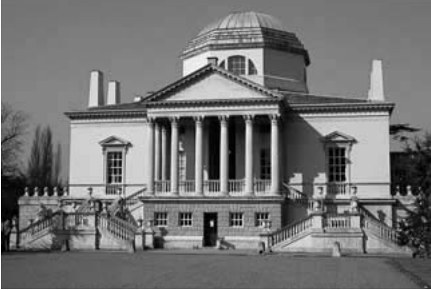
Figure 4.4 Chiswick House exterior showing the central dome admitting daylight. (Photographer Derek Phillips)
