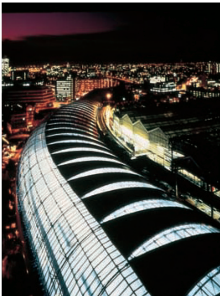
Aerial view at night of the roof structure (Photography Zumtobel).
