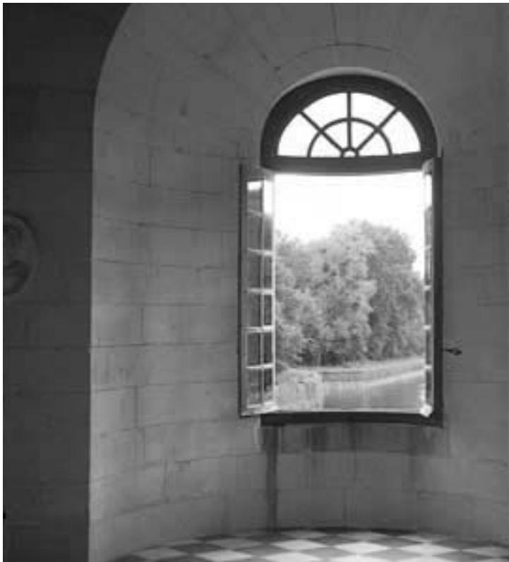
Figure 4.5 The bridge at the Château de Chenonceau in the Loire where daylight is introduced to the interior by the curved window embrasure, reducing the contrast between the inside and the outside. (Photographer Derek Phillips)
