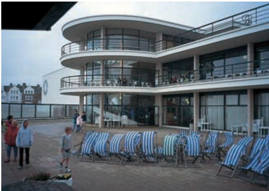
Exterior showing the central staircase (Photographer Derek Phillips).
