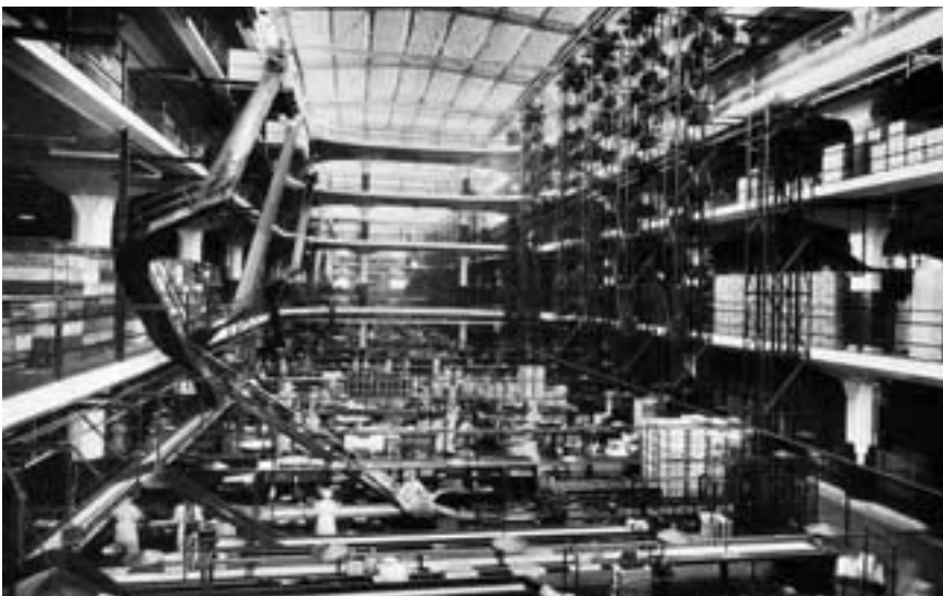
Interior of the packing hall, 1933 (Copyright Boots).
